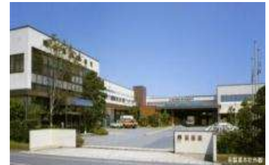
Kotobuki Seika Co., Ltd., Main Plant
