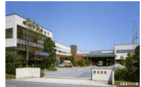
Kotobuki Seika Co., Ltd., Main Plant
